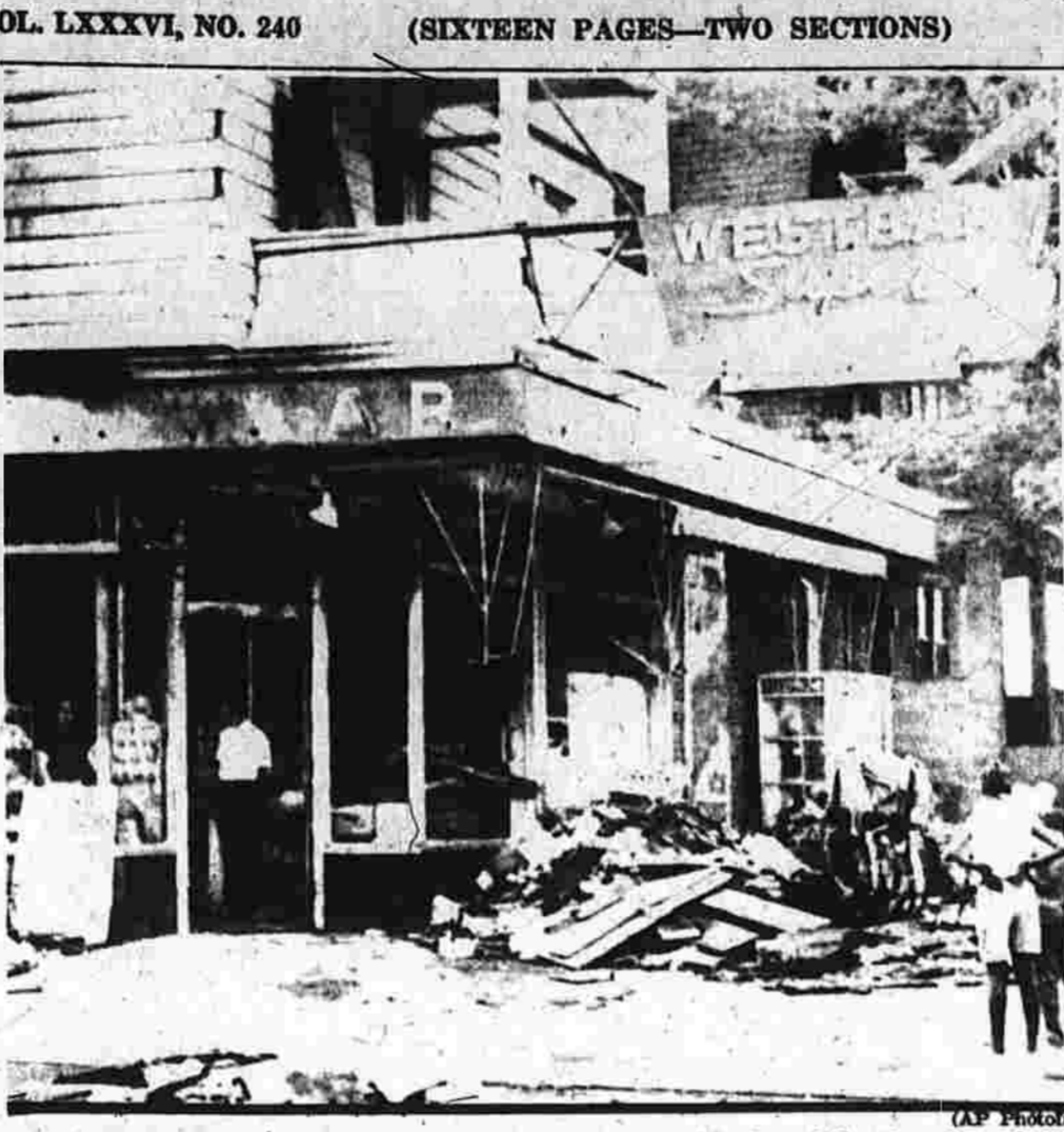
Debris is piled outside Hartford's Westbar Super Market following fire damage. Six business establishments were damaged last night and early today.
